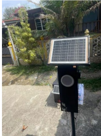
Figure 4. Physical deployment of the smart crosswalk prototype on campus for real-world testing
